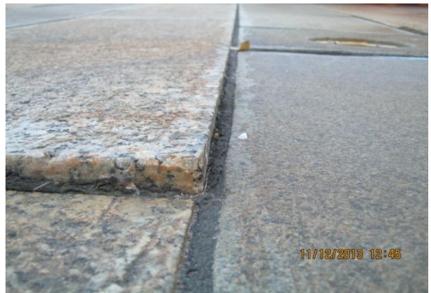
Misalignment of pavers
