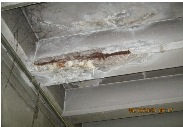
Interior water damage
