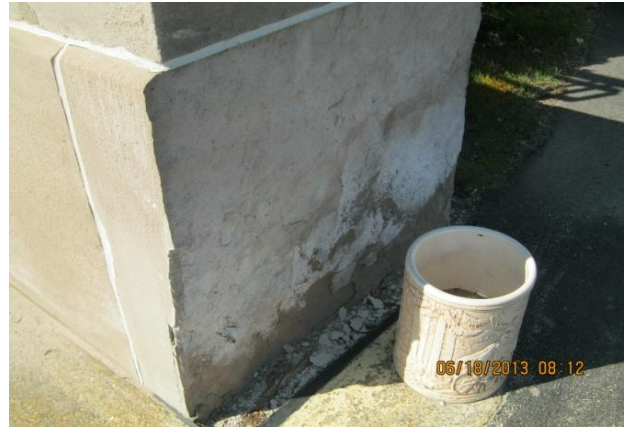
Limestone façade water damage
