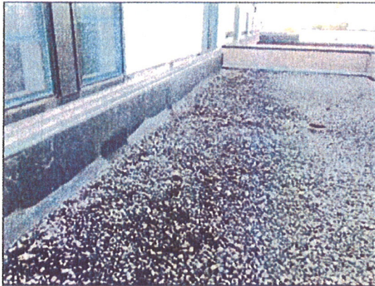
Membrane shrinkage on RA 7
