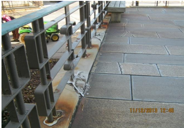
Water damage at failed sealant joints
