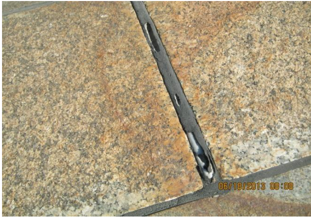
Joint sealant failure
