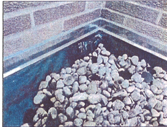
Flashings tenting on RA 7
