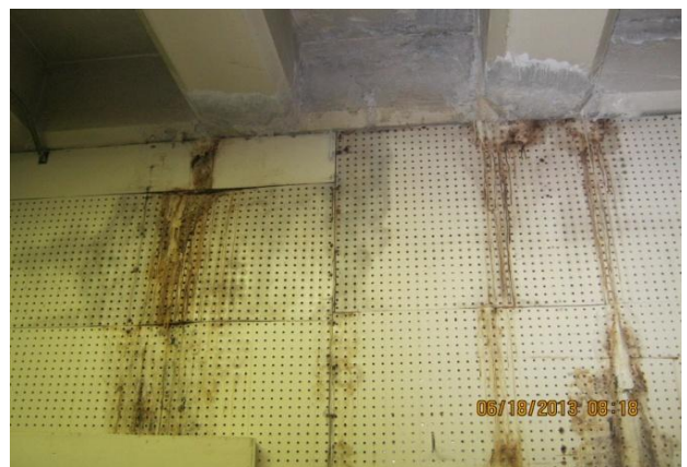
Interior water damage
